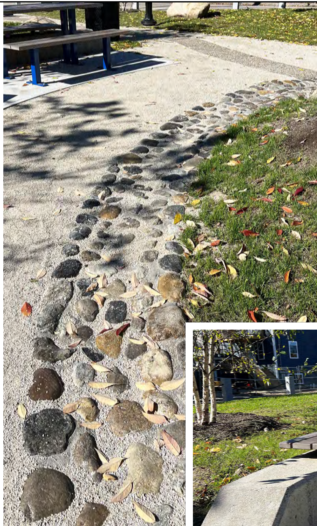
Several Design Details: the exposed aggregate 'River' to represent water since it was not practical to make a new water feature, Cobblestone gutter made from locally-sourced rounded riverstones in mortar to collect water and direct it towards the Raingarden, the radius seatwall featuring a limestone coloring and a sandblasted finish with custom DuMor picnic tables that match the curve of the wall and benches that mount directly to the top of the wall (left to right)
