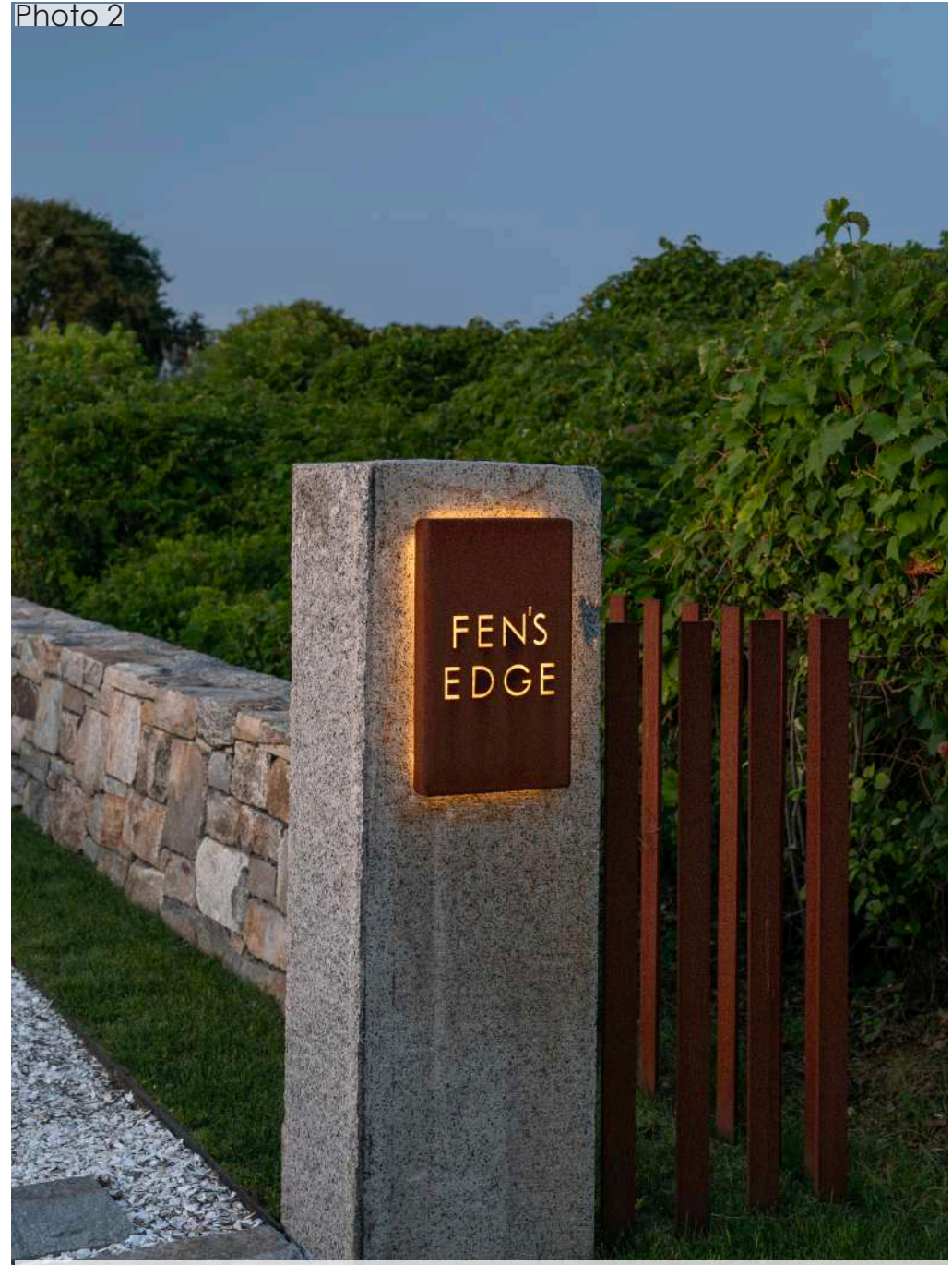
Detail of reclaimed granite posts with corten plaques at dusk.
