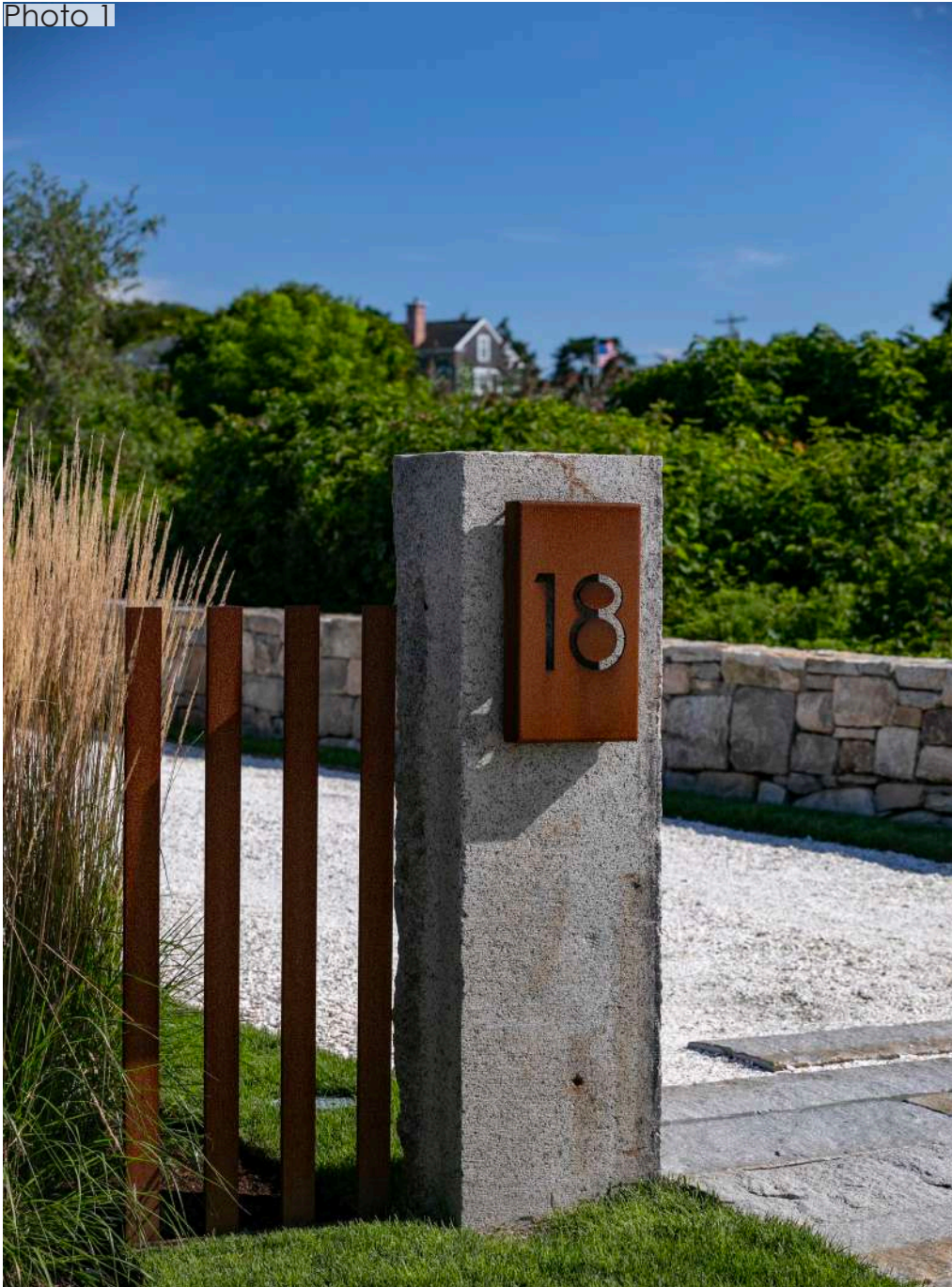
Detail of reclaimed granite posts with corten plaques. *Anthony Crisafulli Photography
