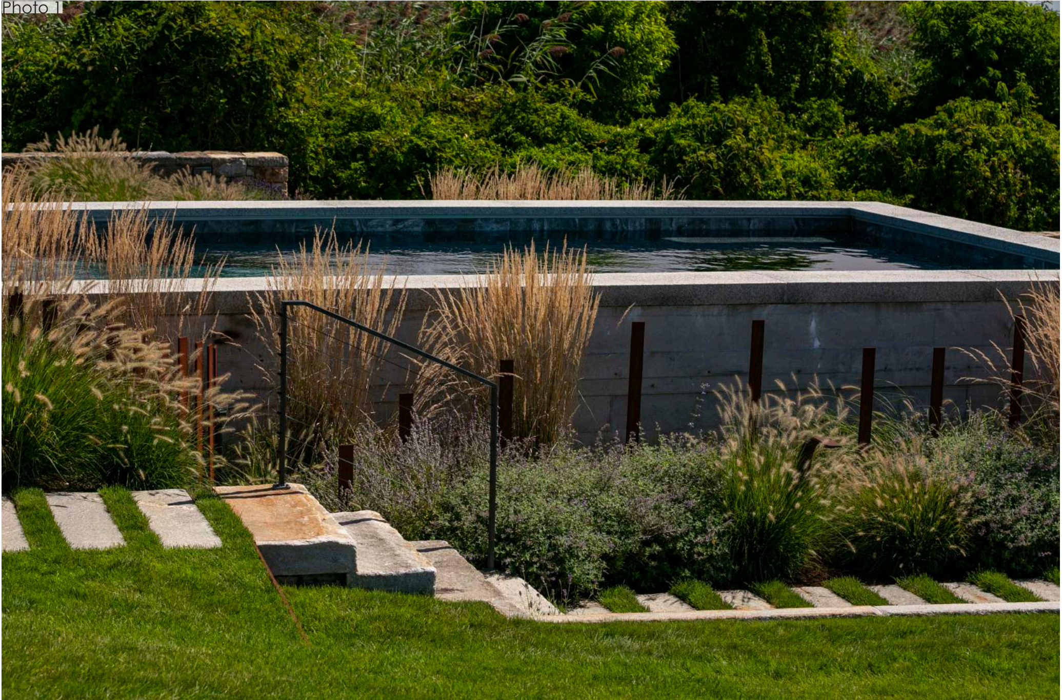
Detail of corten installation. Also shown: board form concrete, pool, reclaimed granite steps, planting.
