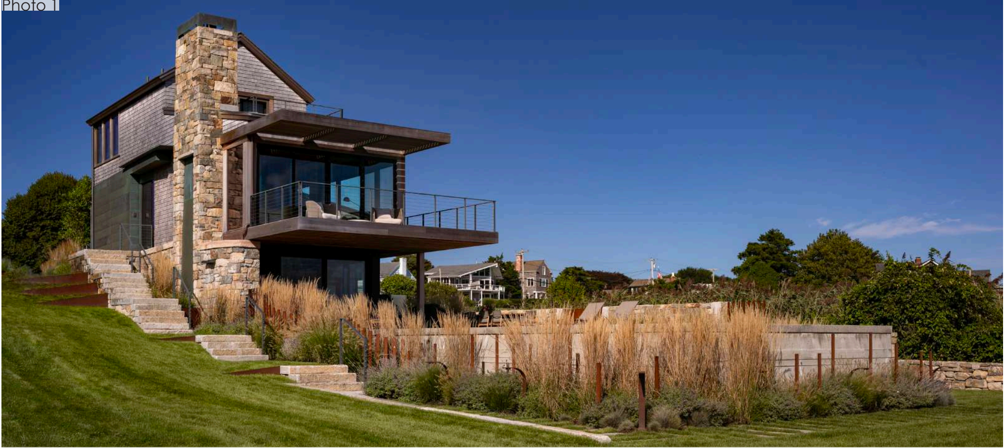
New house, reclaimed granite steps, corten retaining walls, corten installation, board formed walls, lighting, stone walls, planting.
