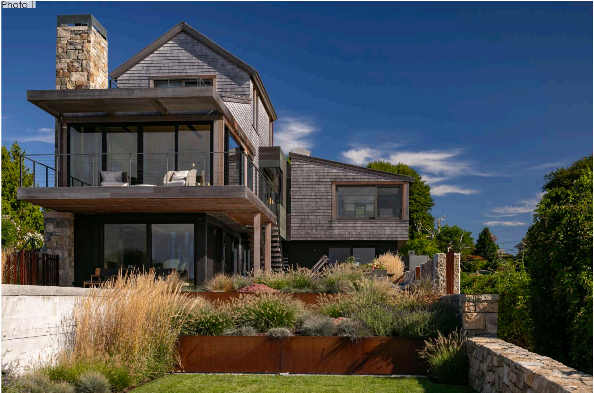
Detail of terraced corten planter beds. Also shown: board form wall, corten fencing, stone walls.
