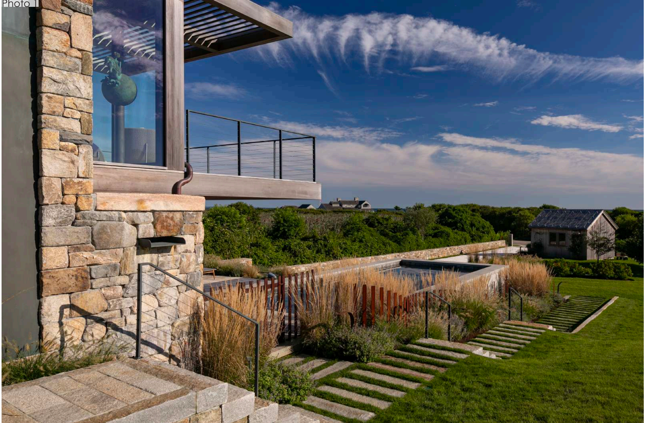
New house, reclaimed granite steps, corten fence and gate, corten installation, lighting, pool, new garage, driveway, planting.
