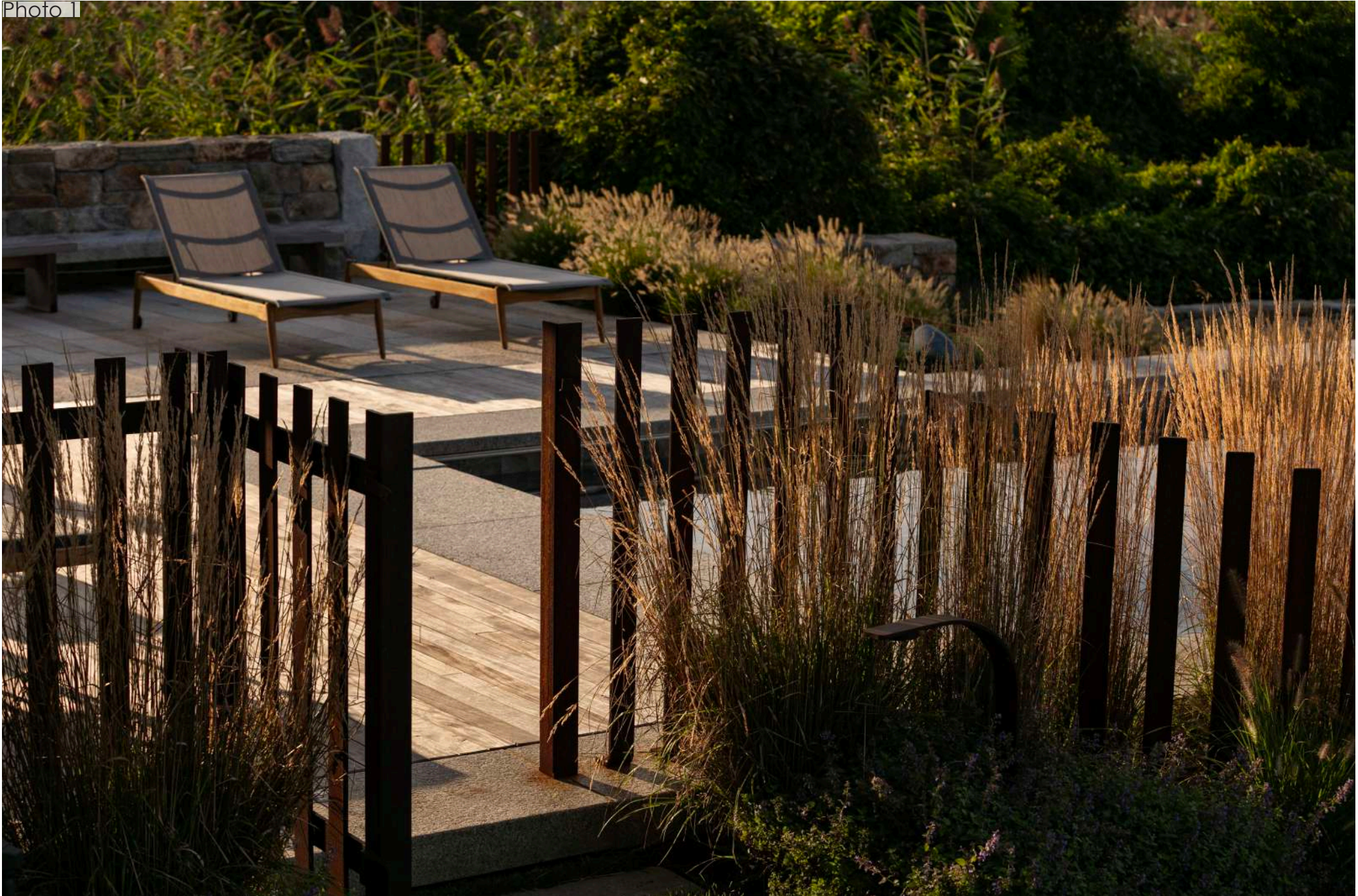
Detail of corten pool enclosure fence and gate. Also shown: ipe decking, granite coping, walls, reclaimed granite bench, lighting, planting.
