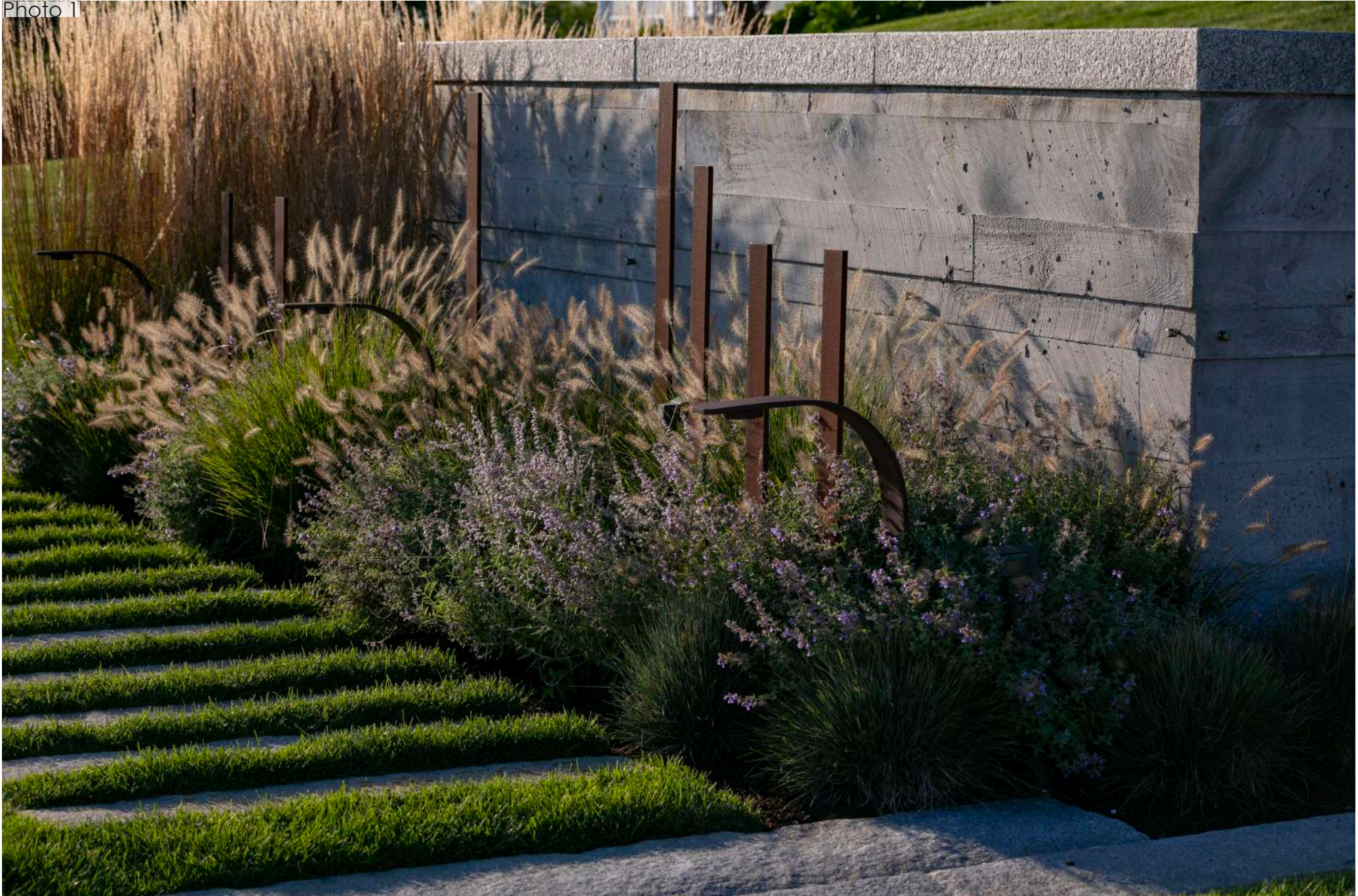
Detail of corten installation and lighting. Also shown: board form concrete, pool, reclaimed granite steppers, planting.
