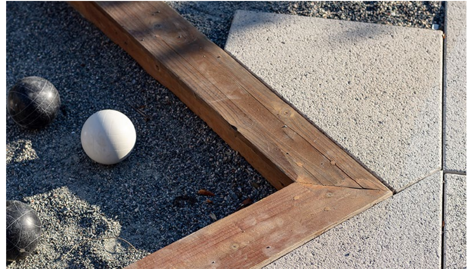
Corner detail for oversized concrete pavers meeting cedar bocce framing.
