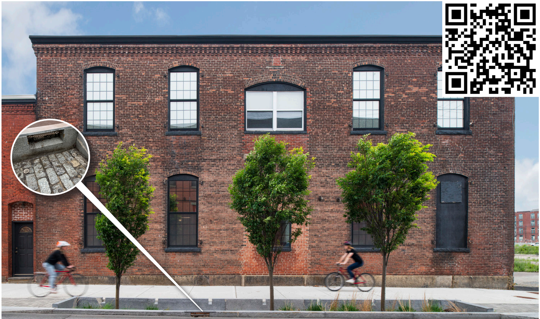
Green Infrastructure Biofiltration Planters Installed. The QR code links to the Pretreatment Operations and Maintenance video.
