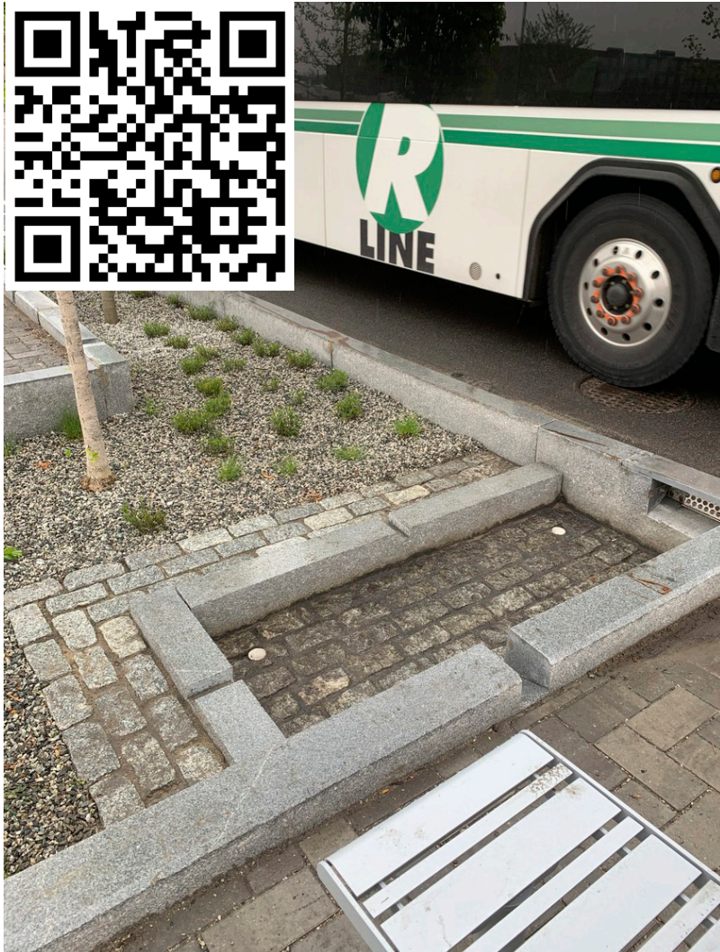
Green Infrastructure Biofiltration Planters Installed. The QR code provides a link to the Permeable Paver Care and Maintenance video.
