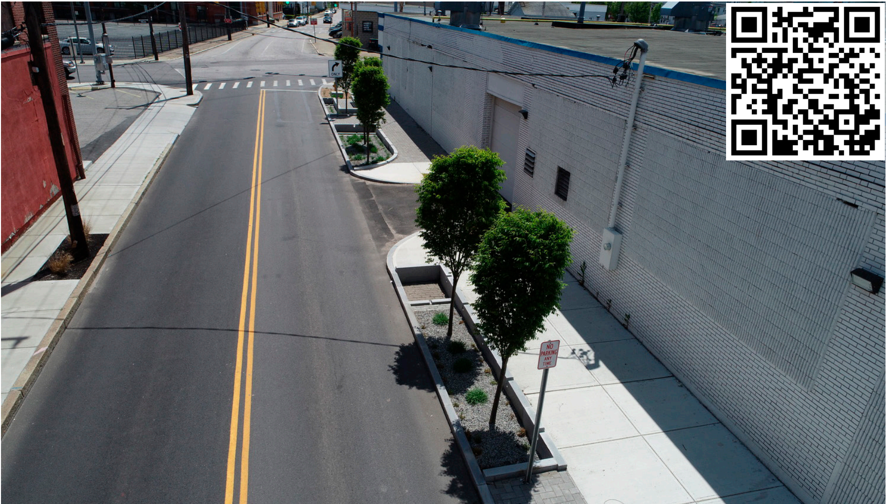
GSI including wider sidewalk, biofiltration planters, and trees for reduction of heat island effect. The QR code link: Overview GI Operations and Maintenance video.
