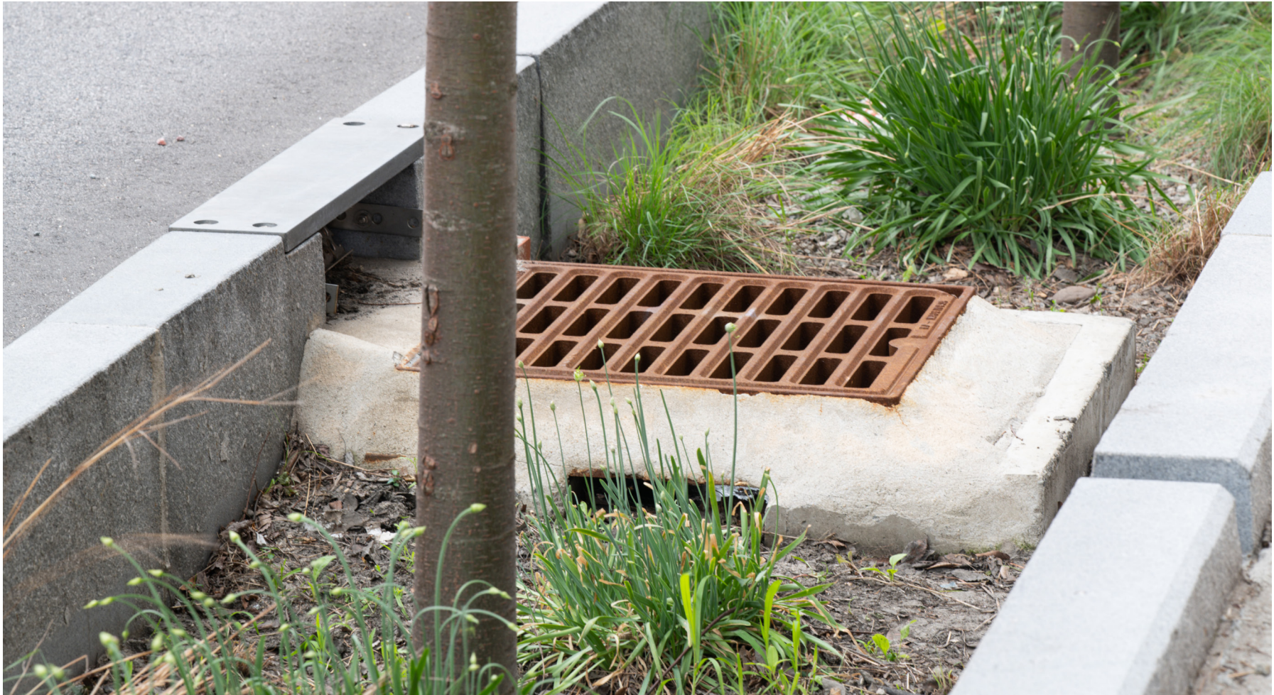
Street trees provide heat reduction. Native forbs and grasses for uptake of stormwater pollutants. Arranged in uniform masses for ease of maintenance. Plantings promote pollination amongst a heavily paved neighborhood.
