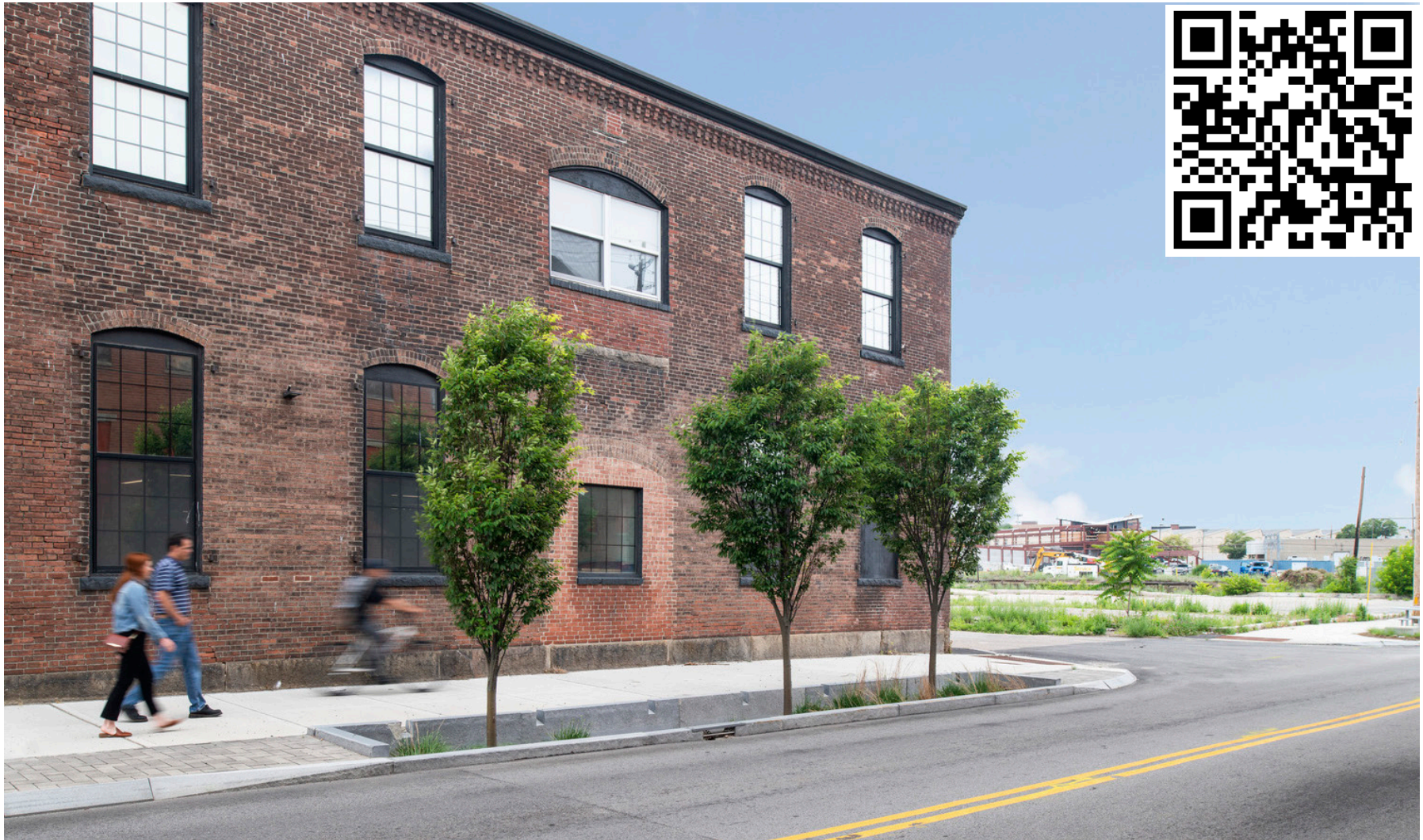
Green Infrastructure Biofiltration Planters Installed. The QR code links to the Planter Bed Operations and Maintenance
